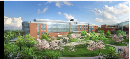
Pre-construction work is underway for the new academic facility for the U.S. Army War College, scheduled for completion in Spring 2023.
