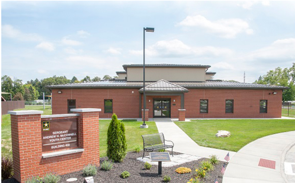
The upgrades will require CDC operations to shift to the McConnell Youth Center, located at 459 Bouquet Road starting Sept. 4 and lasting until Dec. 31.
