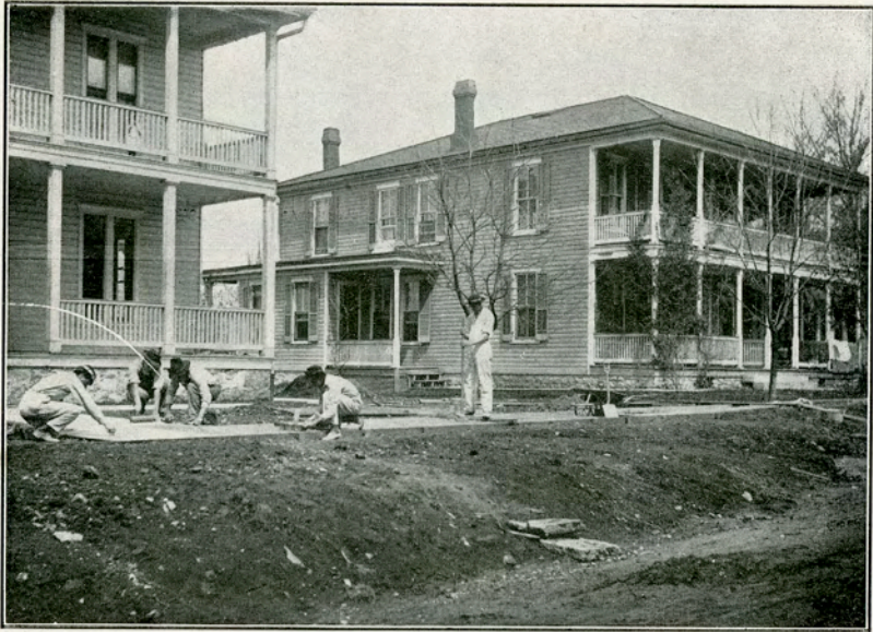
A PRACTICAL LESSON IN CEMENT WALK LAYING.
