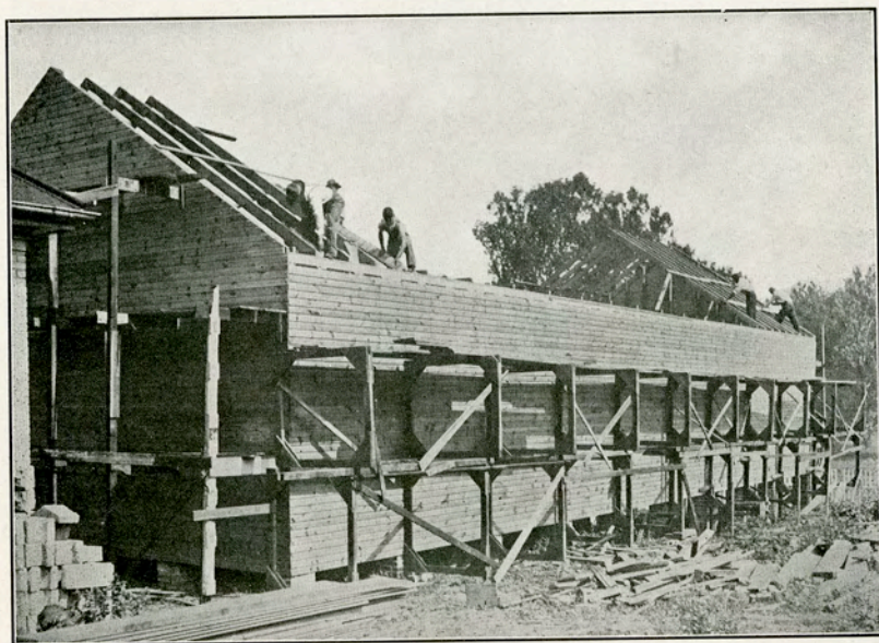
STUDENTS BUILDING A SCHOOL WAREHOUSE.
