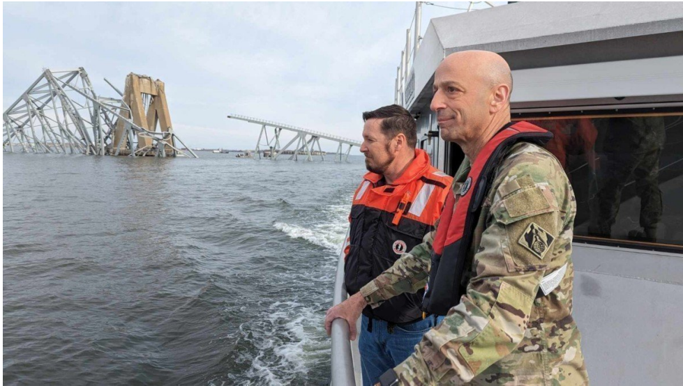
USACE Chief of Engineers Lt. Gen. Scott Spellmon views damage of the fallen Francis Scott Key Bridge that collapsed in Baltimore, March 26, 2024. USACE will lead the effort to clear the channel as part of the larger interagency recovery effort.
