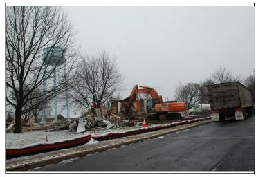
Contractors for Balfour Beatty tear down Smurf houses on Carlisle Barracks Jan. 16. Demolition of the 60-year-old houses should be finished by March and construction will start on more effective and efficient homes. Photo by Tom Conning.
